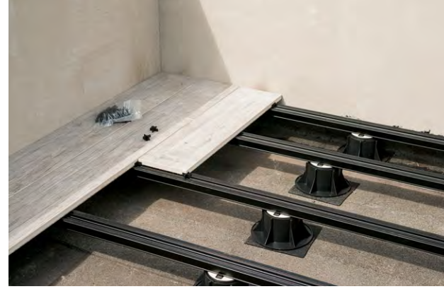
STEP 3 Start laying down tiles from the corner.
