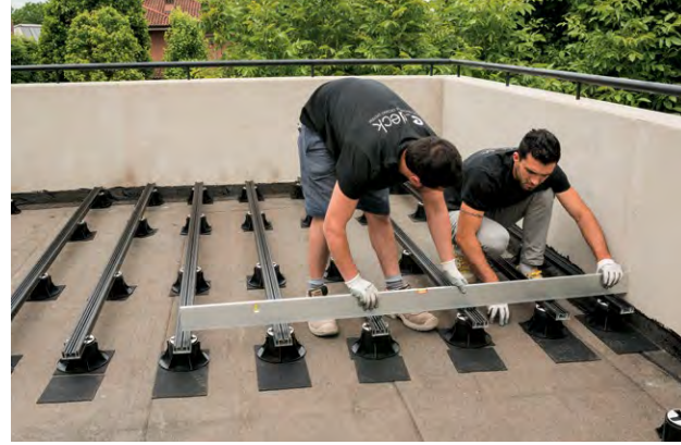
STEP 2 Put the joists into position (12" in-between) and secure them by pressing them down gently.
