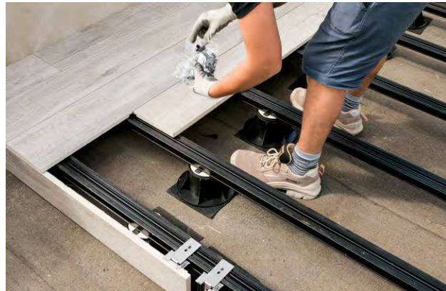
STEP 4 Use the spacers from the kit, in order to lay down the tiles properly.
