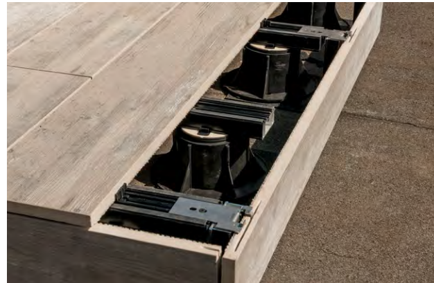
STEP 5 Fix the lateral closure by using the special lateral restraint.
