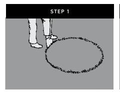
For a lawn, mark a 58" diameter circle with marking paint then go to step 2. For a patio, use chalk instead of paint then skip to step 5.
