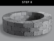
Lay the third layer the same way you laid the second. The third layer joints should line up with the first layer joints. Adhere the blocks with concrete adhesive as you did in step 7.
