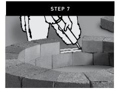
Attach the two layers of blocks together using concrete adhesive. Remove one top block and lay two liberal beads of adhesive near the center of the block. Place block back and press down firmly. Repeat for all 2nd layer blocks.
