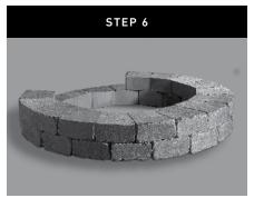
For the second layer of blocks, center the middle of each block over the joint made between the sides of the two blocks underneath it. Place blocks firmly together and level as before.
